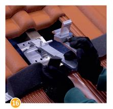
Insert the roof hook into the base plate.
