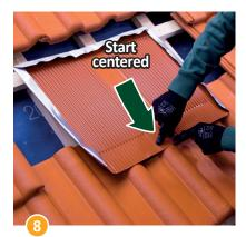
Starting from the center and working outwards, press down the Beta-Plate firmly and ensure it is form-fitting the tile below.
