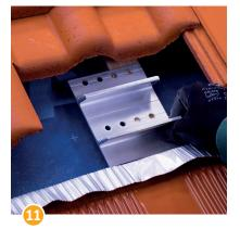
Align the base plate of the roof hook on the rafter.
