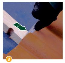
Determine the height of the tile (HT) to be compensated for.
