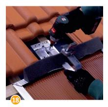
Fixate the positon of the roof hook by tightening the bolt (6 Nm).
