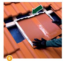
Position the opening of the support plate on the upper batten.
