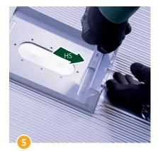
Height of tile (HT) = height of support plate (HS).
