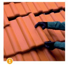
Remove the tiles in the installation area (max. 3 tiles). Position the remaining tiles...
