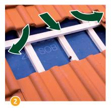
...under the top row, so that the cross battening is easily visible and accessible.
