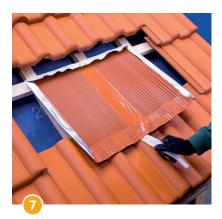
Completely peel off the cover of the adhesive tape from the back of the Beta-Plate.
