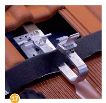
Place the cut of the foam wedge around the roof hook.
