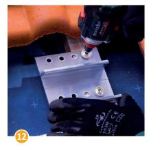
Fasten the base plate to the rafter with a minimum of 2 wood screws ( at least 1 screw per horizontal row of holes) with a tightening torque of 10 Nm.
