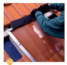
Attach the foam wedge to the rear edge of the Beta-Plate.
