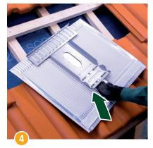
Adjust the height of the Beta-Plate by folding the support plate on the back.
