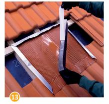
Peel off the cover of the adhesive tape from the back of the foam wedge.
