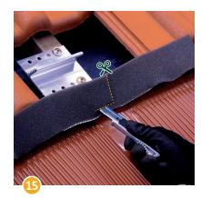
Cut the foam wedge at the position of the roof hook with an L-cut.
