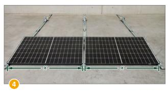
**Installation with corner clamping:** The center distance of the Basic Frames is the module dimension (x) + 22 mm.
