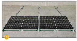
Installation with corner clamping: The centre distance of the Basic Frames is the module dimension (x) + 22 mm.
